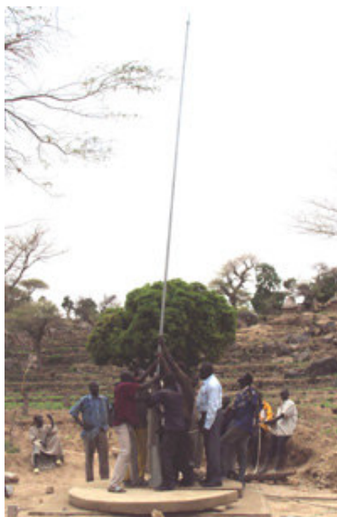
Installation der Pumpe in Ngoshe
